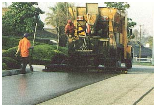
Figure 3- Slurry Surfacing Truck
