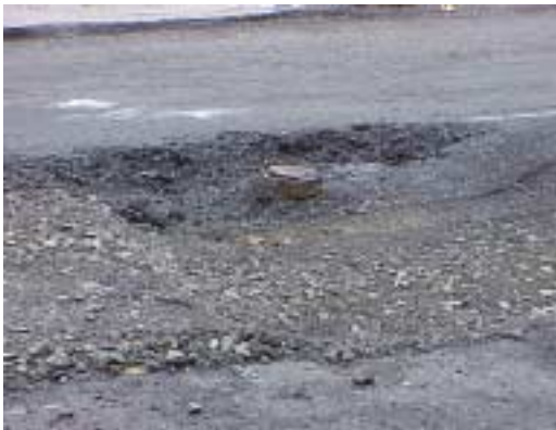
a) Pre-Milling around Utilities
