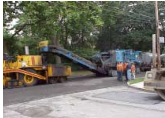
b) In-place Recycling
