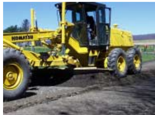
b) Grading with Motor Grader
