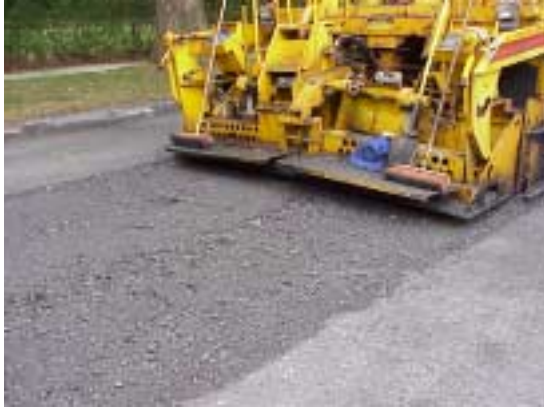
c) Paving with Hot-Mix Paver
