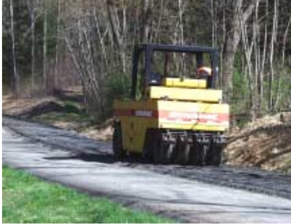
c) Compaction w/ Pneumatic-Tired Roller
