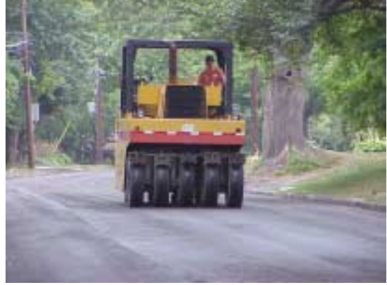
d) Compaction w/ Pneumatic-Tired Roller
